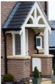
A meter box sited discretely within a porch enclosure.
